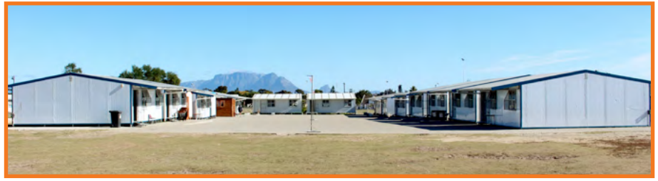
Soneike High School in Kuils River consisting of temporary mobile units.
